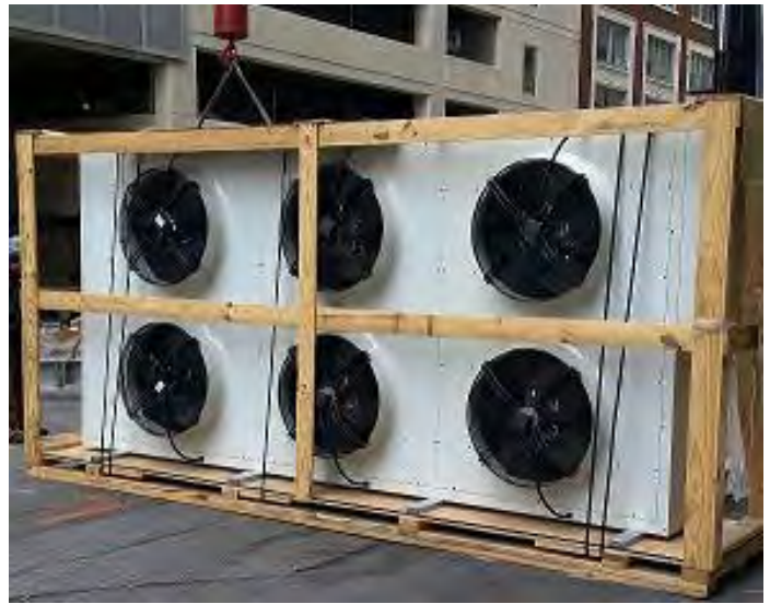
The Data Center dry box as it is about to be craned into position. The dry box is a critical component in the cooling system of our I.T. equipment and allows Commerce to reduce energy consumption.
